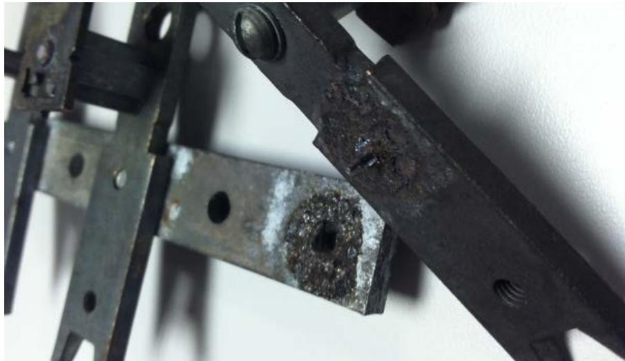
*This is a failed, high-resistance, busbar connection inside a 200 ampere Stab-Lok panel. The arced-away steel screw holds the copper bar in the forefront to the aluminum bar in the background.*
