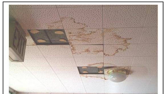
A stained ceiling indicates that water damage has occurred. The source of the water damage should be found and appropriate repairs made.
