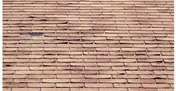
These asphalt shingles are missing, cupping, and blistering. The condition of this roof poses an increased potential of water damage to the interior of the building. Adequate repairs should be made by a qualified roofing contractor.
