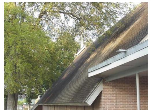
This photo is an example of a tree that should be trimmed back to prevent damage to the roof. Over time, the tree could eventually rub a hole in the roof, allowing water to penetrate the building.
