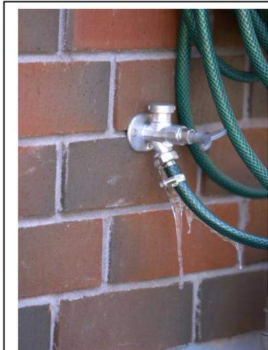
This is an example of a garden hose that should have been disconnected before freezing weather occurred. A building's water line could burst if a garden hose is left connected when the temperatures dip below freezing.
