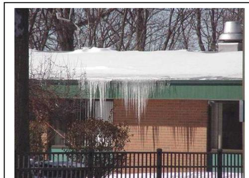
The formation of icicles is a good indicator that there is poor insulation/venting in the attic area. This can lead to water damage.
