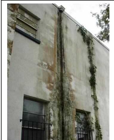
This photo illustrates a missing downspout. The water damage to the building includes algae growth and cracks in the block walls. Regular inspections looking for missing downspouts would have prevented this condition.
