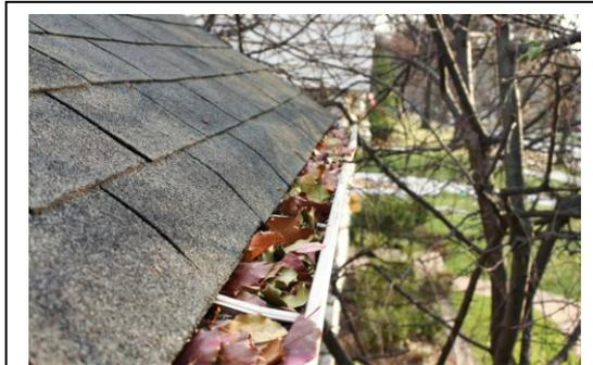
To effectively remove water from the roof, gutters need to be kept clear of debris. This photo shows clogged gutters; water will overflow when gutters are not kept clear of debris.
