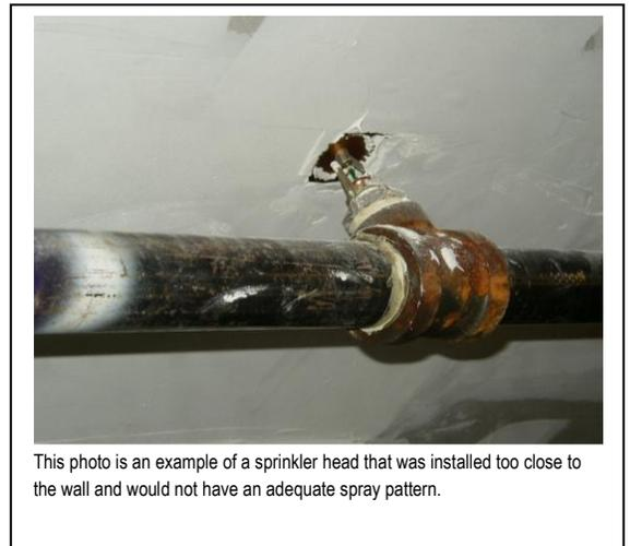
This photo is an example of a sprinkler head that was installed too close to the wall and would not have an adequate spray pattern.
