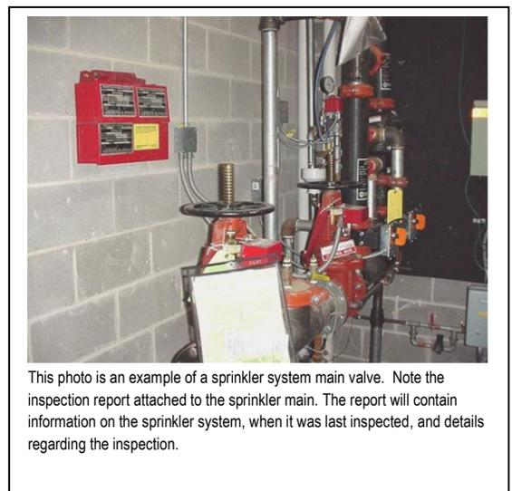
This photo is an example of a sprinkler system main valve. Note the inspection report attached to the sprinkler main. The report will contain information on the sprinkler system, when it was last inspected, and details regarding the inspection.
