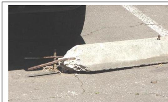
This photo illustrates a severe trip hazard due to the exposed rebar from the deteriorated tire stop. If a trip and fall would occur here, the potential for a severe injury is present from the sharp and exposed rebar rods. To correct the hazard, the entire tire stop should be replaced.
