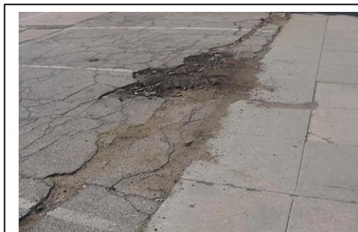
This photo illustrates a parking lot that has deteriorated creating trip and fall hazards due to the numerous cracks and depressions in the surface. To correct this hazard, the sections of asphalt should be resurfaced.
