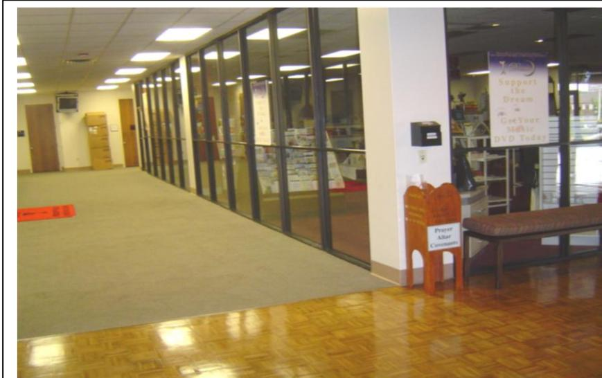
This photo shows a difference in flooring surfaces from carpet to wood tile. Potential slip and fall hazards exist due to the different flooring surfaces installed in a common pathway. Ideally, the surfaces should be consistent. Also note the high degree of smoothness to the hardwood flooring, which also could lead to a slip and fall.
