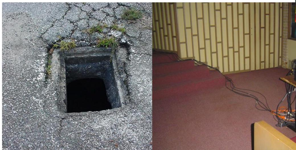
The photo on the left shows a **drainage hole** that should have a protective covering installed. The photo on the right shows **electrical and audio cables** placed on the stairs and walking surface that should be routed away from the walking area, taped to the floor or provided with cord protectors. Areas such as these create unnecessary trip and fall hazards and should be corrected.
