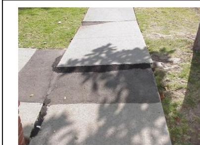
This photo illustrates severe trip hazards due to the uneven walking surface. Patching has been completed; however, it is not adequate. In this case, the entire section of the sidewalk should be replaced.
