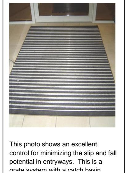
The best design consists of a **grate system** with a catch basin (shown on the right), which is installed at high traffic areas to effectively remove moisture from footwear. If a grate system is not feasible, mats should be installed.
