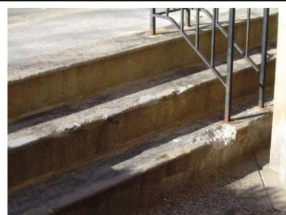
Routine inspections should be conducted to locate and repair any hazards, such as the deteriorating steps in the photo above. Conducting routine inspections and maintenance will help prevent slips and falls from occurring.
