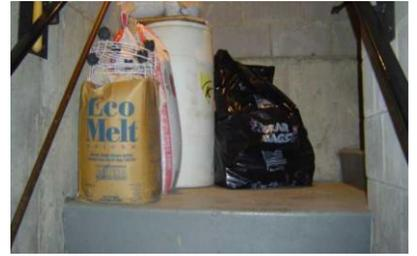
This photo is an example of materials being stored on a stair landing. Storing items on stair landings restricts the walkway, increasing the chances of slips and falls to occur.
