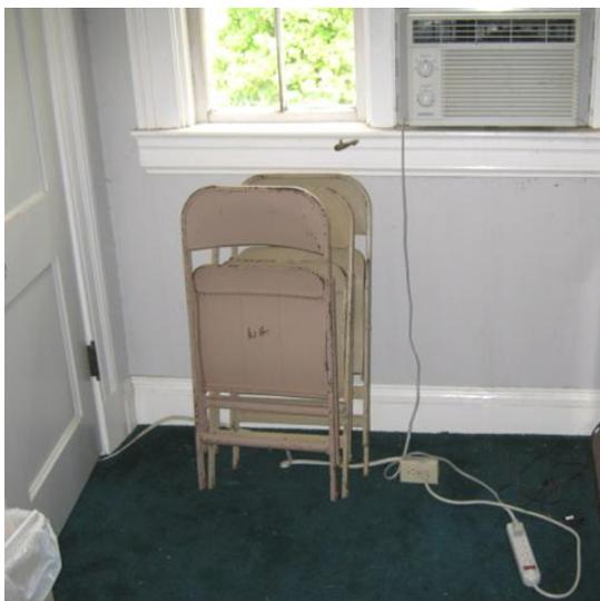
This image shows several wiring hazards; a "homemade" extension cord on the floor that is run under a doorway, which has an outlet installed at the end, that has a power strip plugged into it that is supplying power to a window air conditioning unit. This is a fire just waiting to occur.
