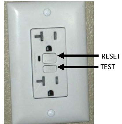
The image on the left shows a standard electrical outlet that is installed too close to a water source. This outlet should be GFCI protected and installed with an outlet similar to the image on the right. GFCI outlets are easily identified as they have a “TEST” and “RESET” button.
