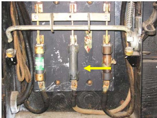
This image shows a piece of metal tube that was inserted in the middle circuit. This is being used as a conductor and was most likely installed because the existing fuse kept blowing. This practice should never be done.
