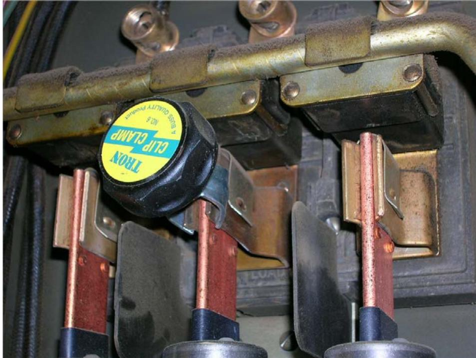
This image shows a clip clamp being used to eliminate the heating that was actually being caused by high resistance connections inside the fuse. The real problem is the clips do not have enough compression and should be replaced (Photo courtesy of Hartford Steam Boiler).
