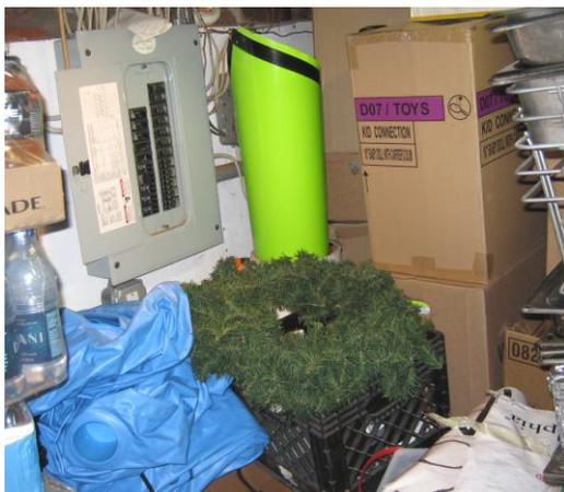
Storage and housekeeping practices next to this electrical panel greatly increase the chances for a severe electrical fire. Note the heavy fire load associated with all of the combustible materials present.
