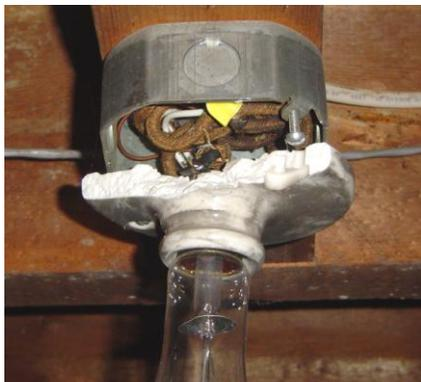
This image shows a broken light fixture. This exposes the wiring to physical damage, dust, dirt and moisture accumulation.
