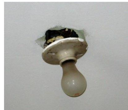
This image shows a light fixture that is unsupported, which puts undue stress on the electrical connections.
