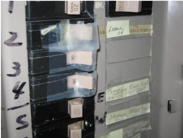
Image above shows breakers taped in the ON position. This practice should never be done.
